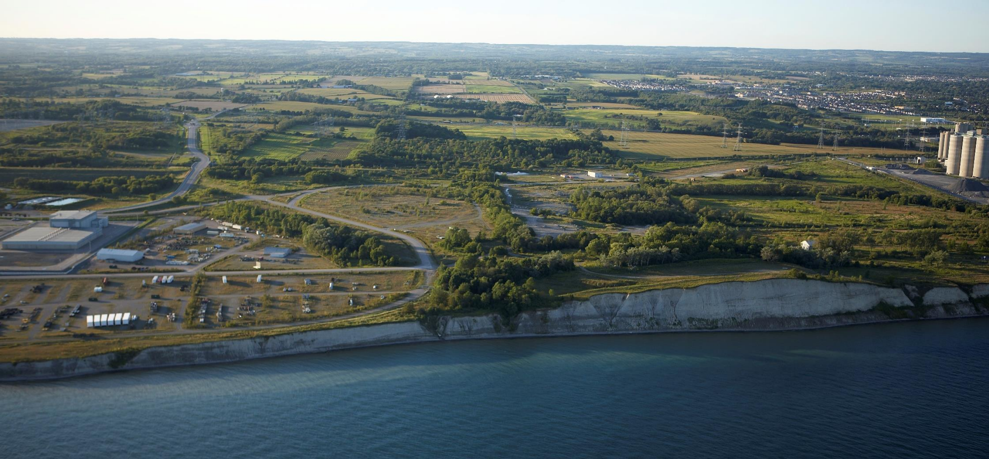
Figure 2: Aerial View of DNNP Project Site Looking North from Lake Ontario (circa 2008).
